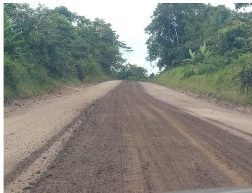
Fig. 1. Road conditions before repair.
