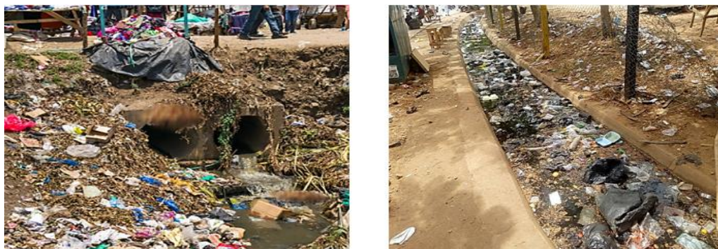
Fig. 4. Impacts of plastic wastes on drainage systems.
